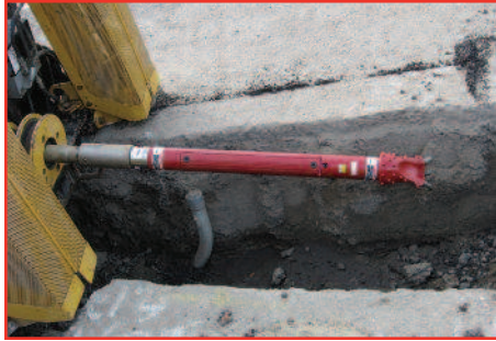
The 4.25" Eagle Claw starting into the first bore, 320' in hard rocky shale.
